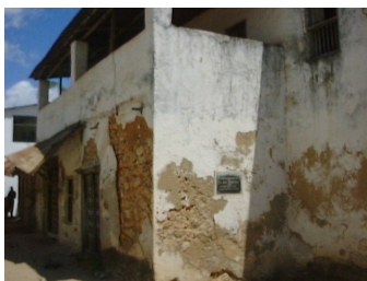
Left: Livingstone House before work commenced.
